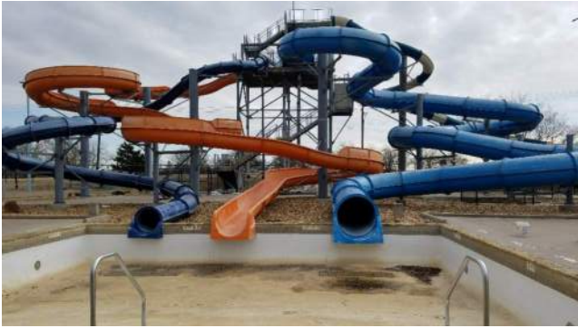
Existing Plunge Pool
