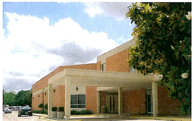
Covered Canopy @ Fellowship Hall
