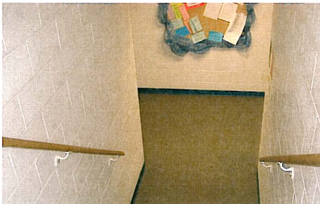
Typical stair / CMU walls
