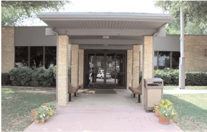
Existing front entry canopy
