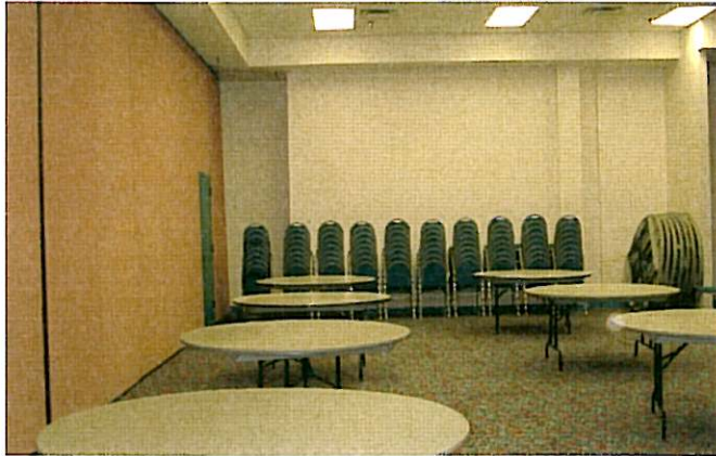
Movable partitions @ Fellowship Hall
