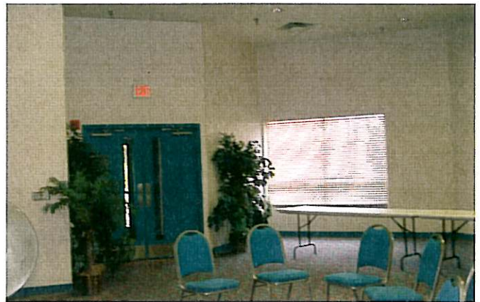
Entry doors @ Fellowship Hall
