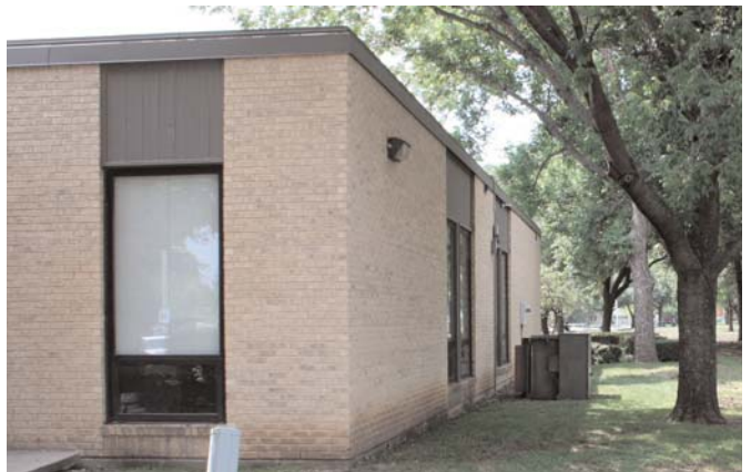
North elevation / Administration area
