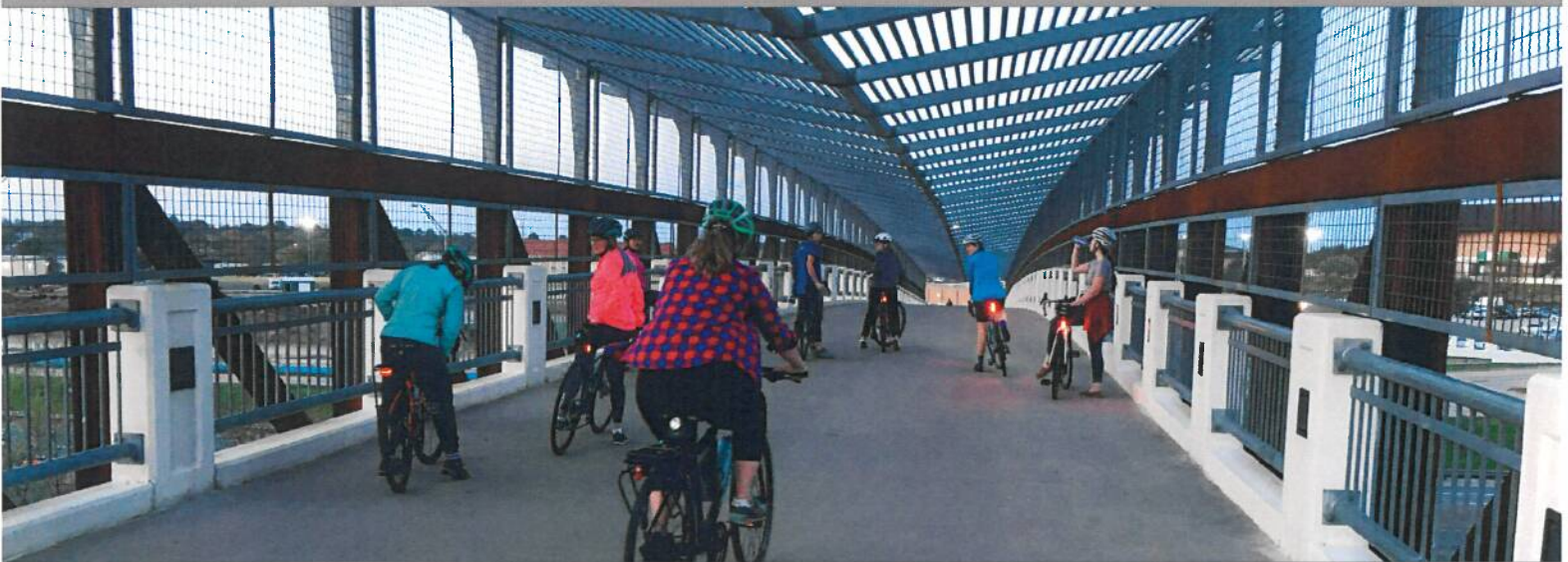
UNT Pedestrian Bridge Photo Credit: Suzanne Rumohr
